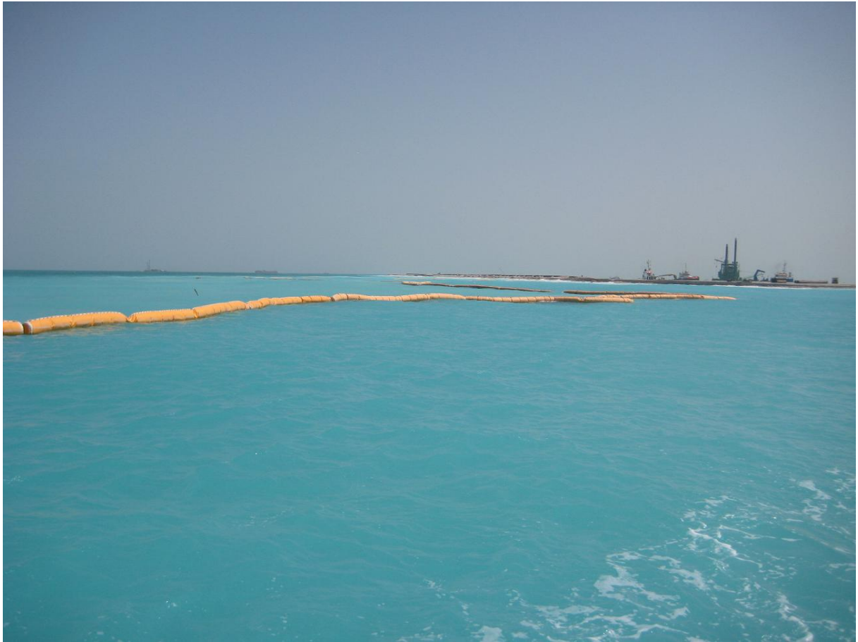
Figure 1.2: Multiple sections of hanging silt screens as applied at a dredging project in the Middle East, courtesy Boskalis.
