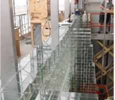
Figure 111. The mast climbing working platform and one of the three mobile elevated platforms (Oikonomopoulou et al., 2017)
