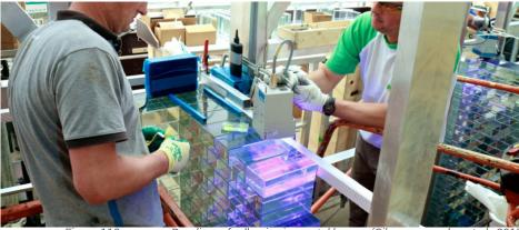
Bonding of adhesive in crystal house (Oikonomopoulou et al., 2017)
