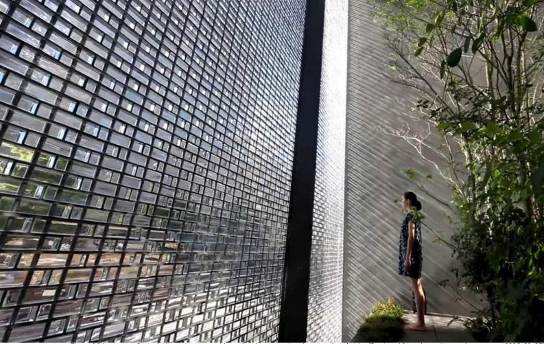
Figure 104. Optical House in Japan with steel rods connecting the cast glass bricks (Retrieved from: https://www.dezeen.com/2013/01/27)
