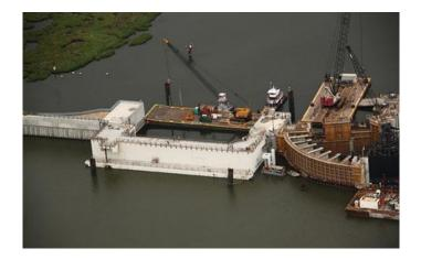
Figure 9-11. Gulf Intracoastal Waterway Floating Barge Gate made of HPLC
