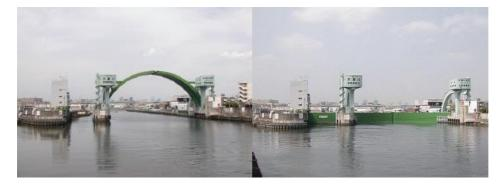
Figure C- 11. Front view of a Visor Gate in Osaka, Japan (Left: open; Right: closed)
