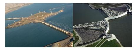
Figure 9- 35. Left: artificial Island in the middle of Eastern Scheldt barrier; Right: chamber of Maeslant barrier built on land
