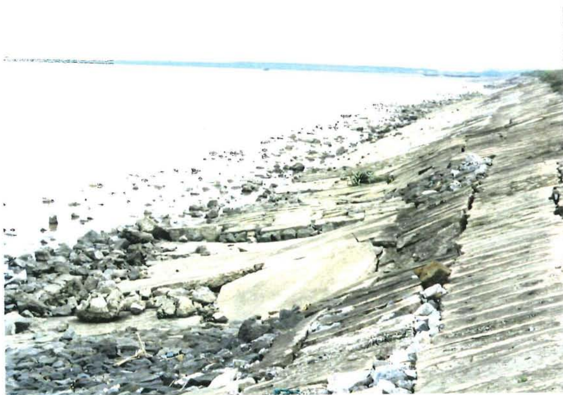
Picture I.7 Damage of concrete grouted stones revetment in Hai Phong Province
