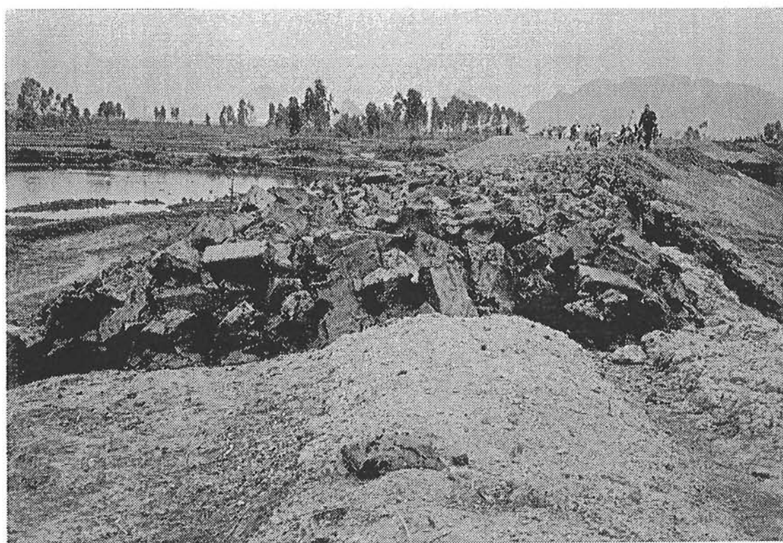
Figure 5.1 Earthfill of clay: difficult to compact
