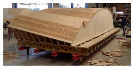
Figure 37. Formwork for a ruled surface, consisting of planks placed on top of a rig. (Bau & Technologie 2006)
