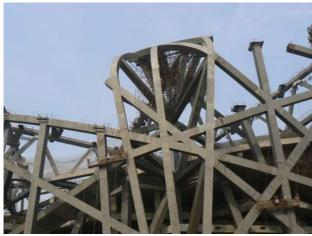
A. Overview of two primary trusses and a secondary beam diagonally running through it.
