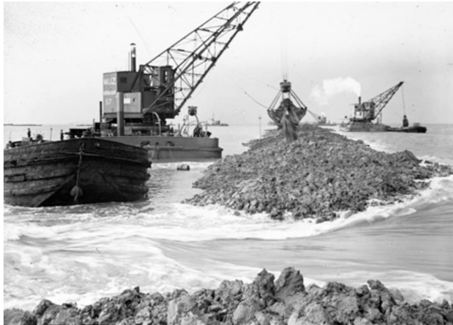
Figure 1.1 Acceleration of flow through a closure gap
