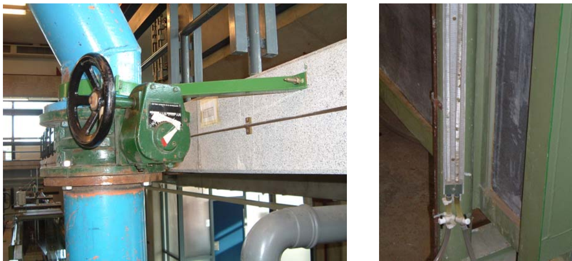
Figure A.4 Inlet valve (left), pressure gauge for measuring the discharge (right)
