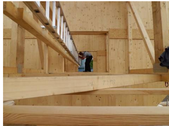
(d) Premounting the ladder in a scaffolding section
