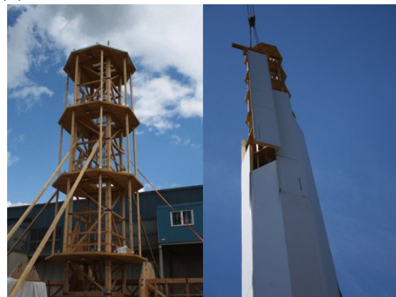
(f) Panels are mounted on the scaffolding
