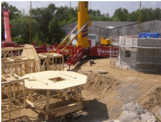
(c) Assembling a scaffolding section on site
