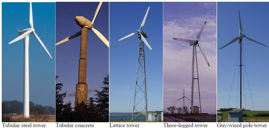
Figure J-1: Examples of different structural systems and materials
