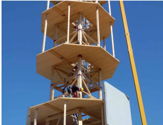
(g) Workers align the next 15 m tall section of the scaffolding
