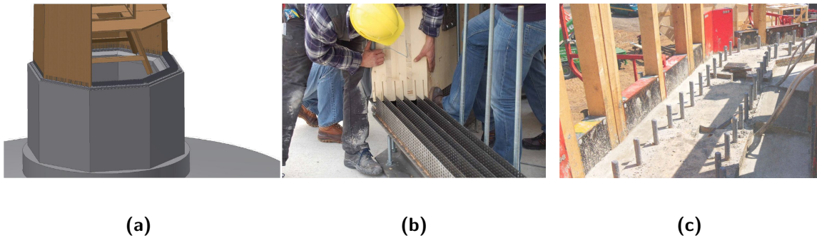
Figure K-8: The connection between base and tower is made by gluing a footplate into the wood (b) and connecting this with anchor bolts (c)
