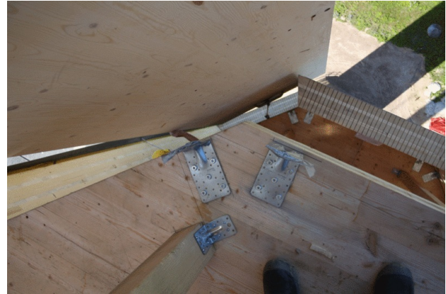
(h) The panels are held into place by the scaffolding until the panel connections have been made
