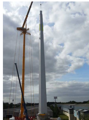
(j) Installing the steel adapter
