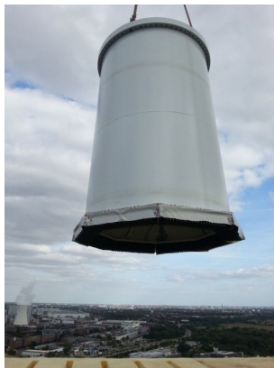
(i) Hoisting the steel adapter to the top
