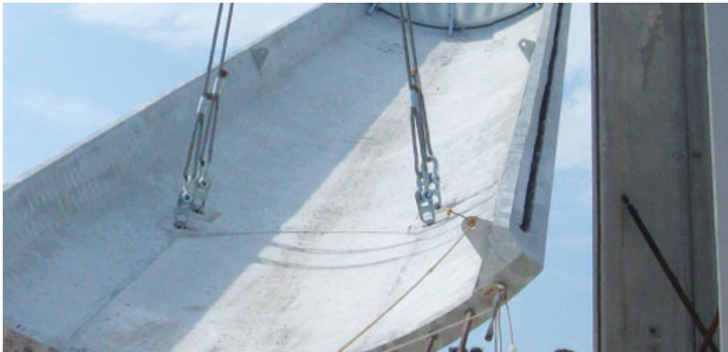
Figure J-6: Close-up of a precast concrete tower section
