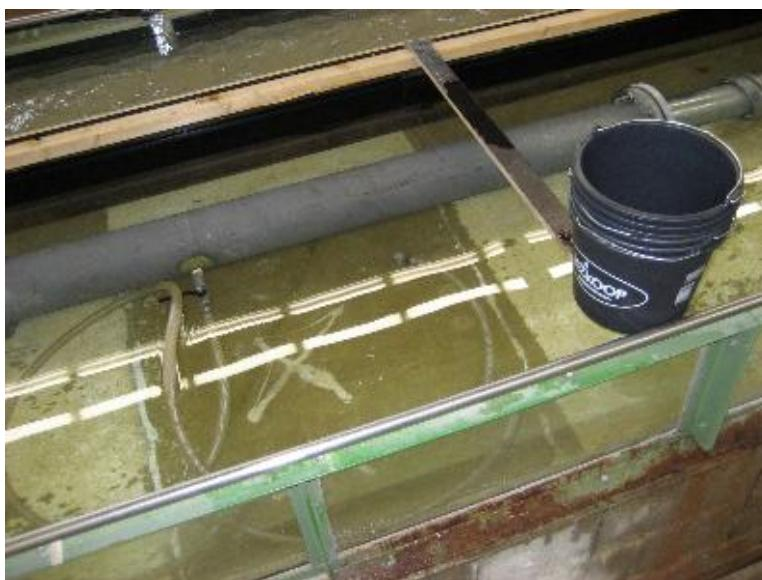
Figure 11 Sediment tap in return pipe
