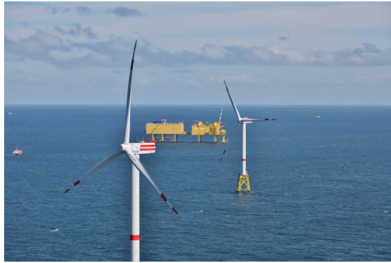
Figure 1: Offshore Wind Substation [3].
