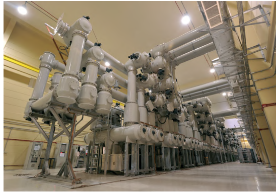
Figure 4: GIS Example [8] inside of a yellow substation in Figure 1
