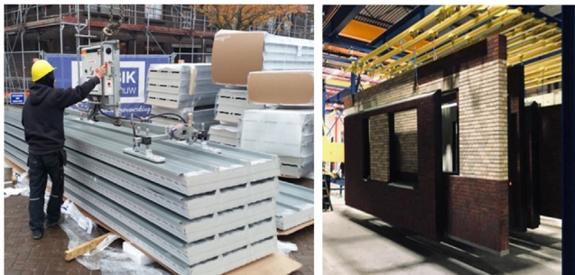
Figure 10.4 (A) Prefabricated roof panels used in the construction of the 12 zero-energy dwellings, in Vlaardingen, the Netherlands. (B) CompletRC RC Panels ( Rc Panels, 2021 ) with weather finishing of brick tiles.
