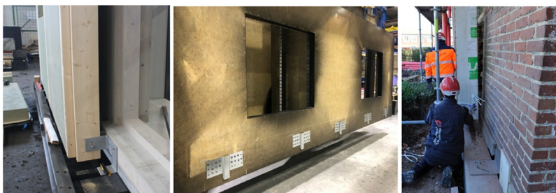
Figure 10.3 (A) The panels are connected to wooden posts, attached to the existing structure with steel U profiles. (B) Anchors on the back of the façade panel, to be connected on rails attaching to the existing building. (C) The installation of the prefabricated panel on the concrete block that bears the extra weight. Hem, France, Net-zero retrofit, under construction, Vilogia.
