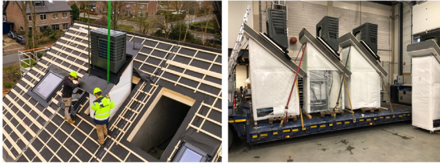
Figure 10.11 Preassembled building services unit placement on the roof. Factory Zero, the Netherlands, energy modules.
