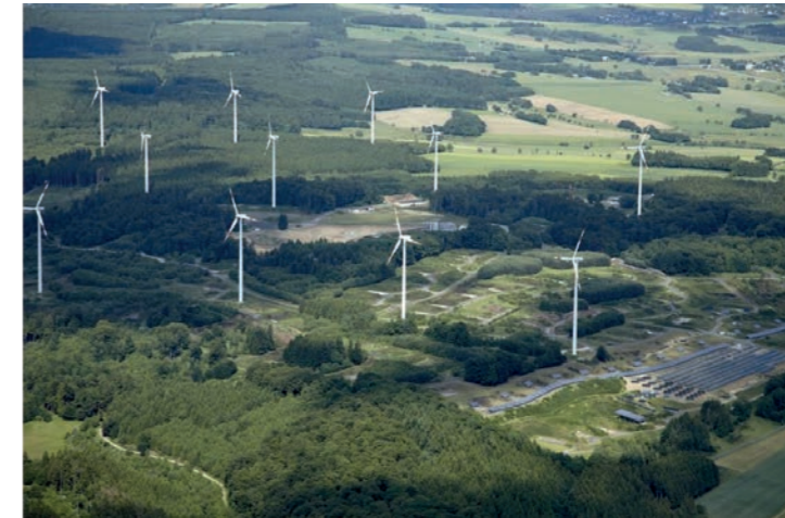
FIG. 2.4 Renewable energy park in Morbach, GE. Source: timbre-project.eu
