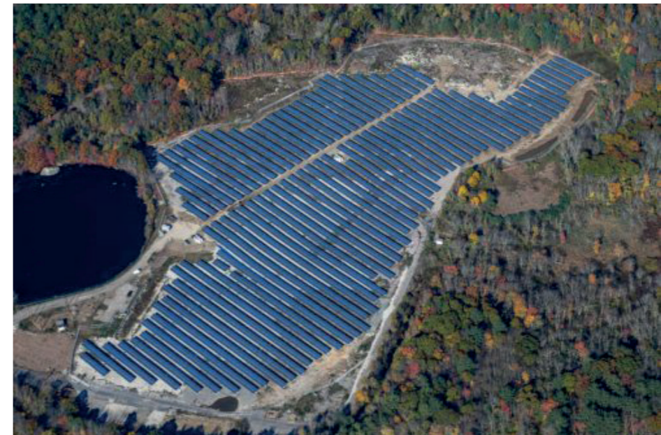
FIG. 1.5 A 4.75-MW solar farm on Brownfield in Massachusetts. Source: Greg M. Cooper / Soltage LLC
