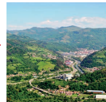
The narrow Caudal valley has created a dense urbanization pattern where housing, industry and infrastructure are tightly packed together. Source: Ayuntamiento de Mieres
