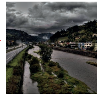
The narrow Caudal valley has created a dense urbanization pattern where housing, industry and infrastructure are tightly packed together. Source: Mapio.net
