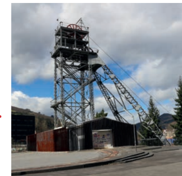
Castilletes, structure to extract coal from the mining shafts. Dozens of these structures can still be seen in the mining valleys. Source: author
