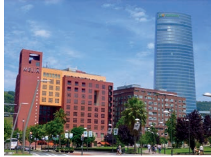
FIG. 4.5 Hotel Meliá Bilbao and Torre Iberdrola on of the succesful project of Bolbao Ria. Source: commons.wikimedia.org
