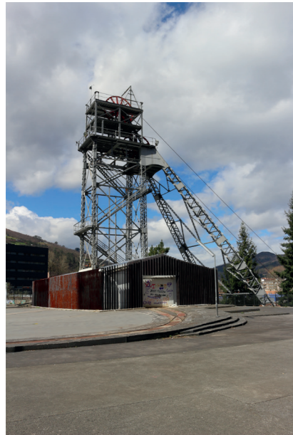
FIG. 3.18 Efforts to valorize the industrial heritage of the mining valleys. Source: author
