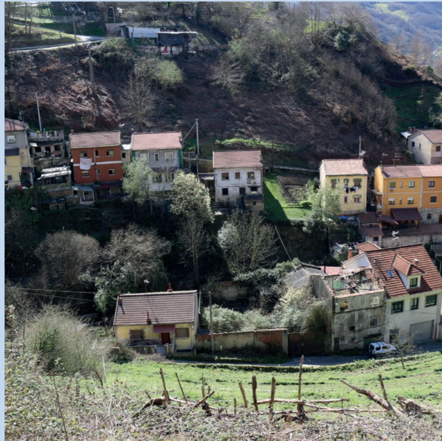
Holes in the urban pattern through neglect and abandonment in Mieres, Asturias. Source: author
