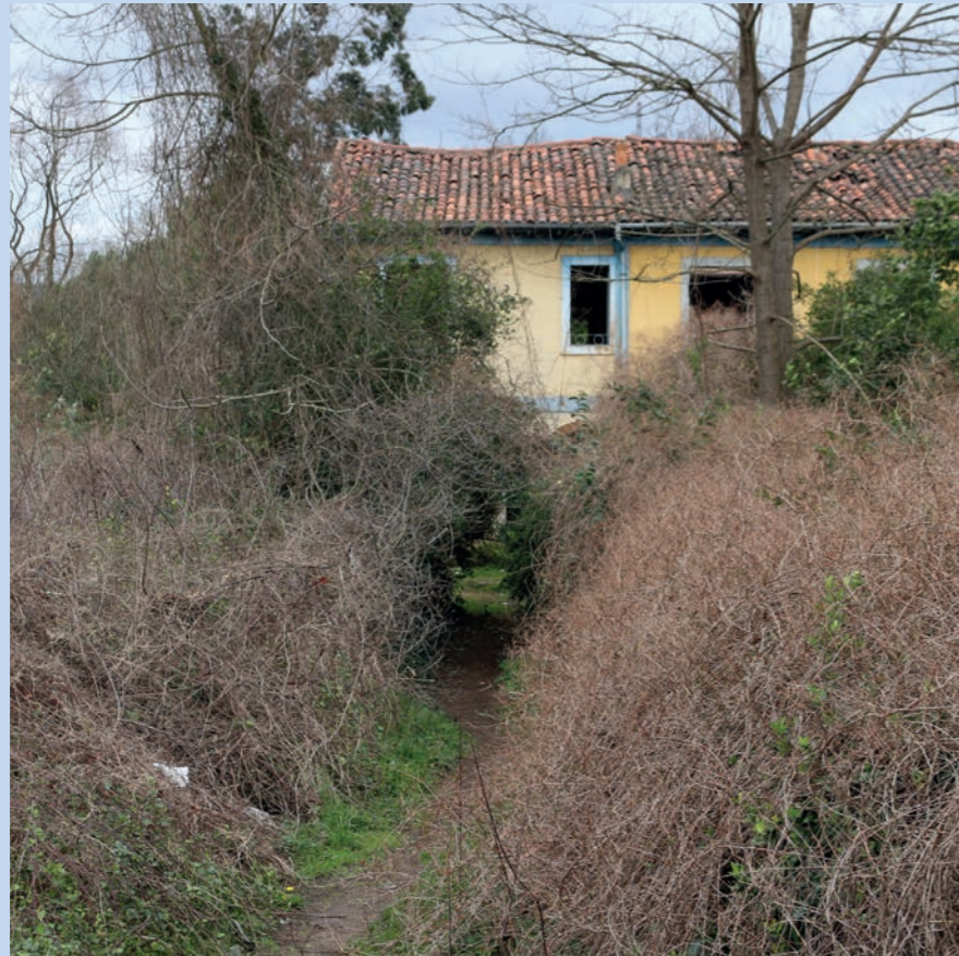
Abandoned house in Langreo, Asturias. Source: author
