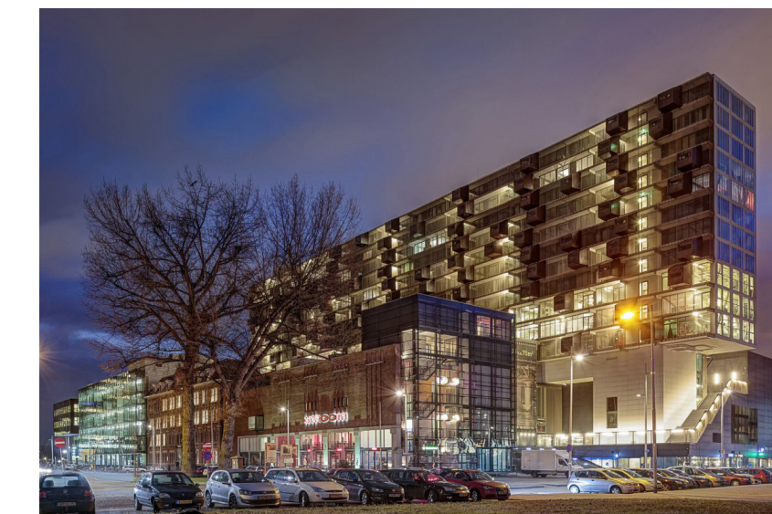
8.2.2 Photographs of the Schiecentrale 4B complex
