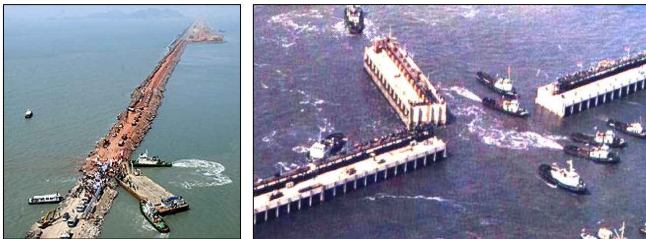
figure O-1: Saemangeum barrier South Korea and caisson closure
