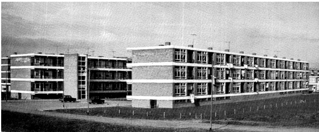
Figure 3: Stellendamhof – a gallery flat in Rotterdam Pendrecht.
