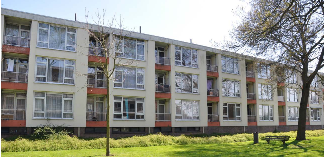
Figure 4: Stellingdamhof –the façade towards the collective garden.
