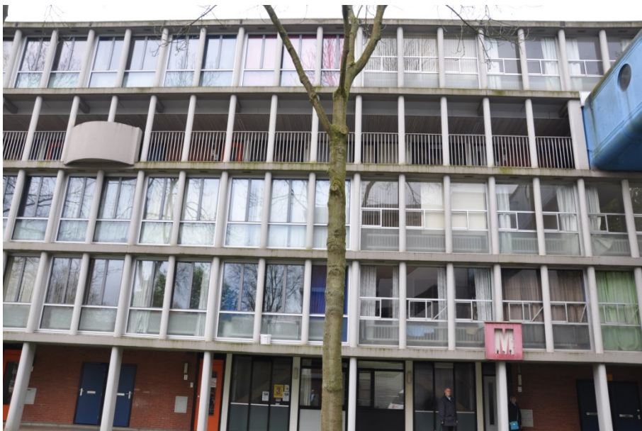
Figure 6: The façade before and after renovation. Left: the new windows, right: the old ones.
