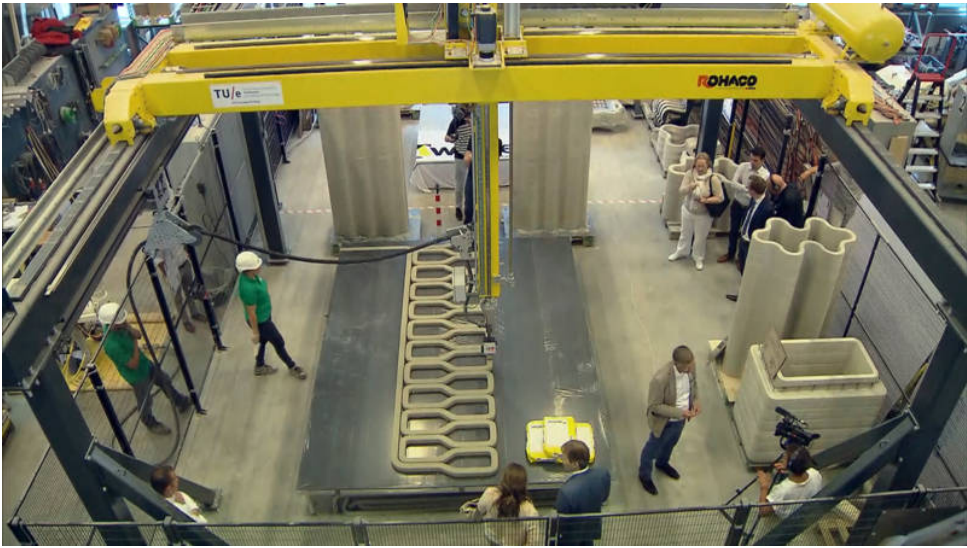
Figure 6.3: 3D-printed structure of Gemert bridge in Tu-Eindhoven, adapted from https://nos.nl/
