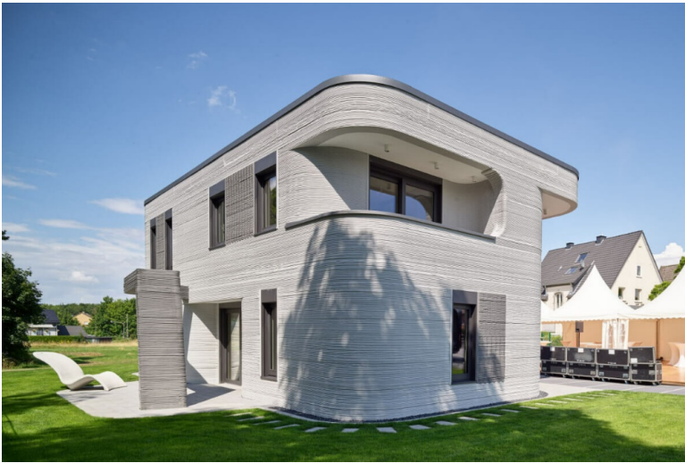
Figure 1.2: A 3DC printed two-story single-family house in Beckum, adapted from ( https://sievert.de )
