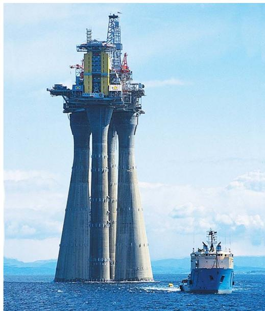
Figure 2.2: Concrete Gravity Based Structure (Troll A platform) [17]
