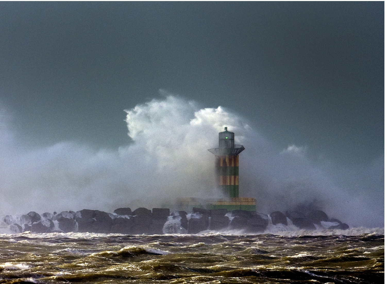
Figure 17: Pier in IJmuiden
