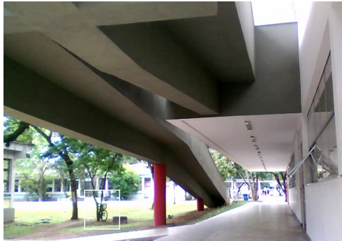
Figure 6 Users appropriate the surroundings for bicycle parking.
