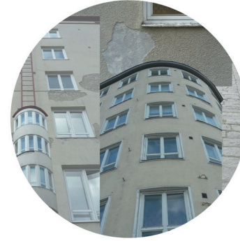
40s to 50s less ornamentation, subtle colours, plastered facades
