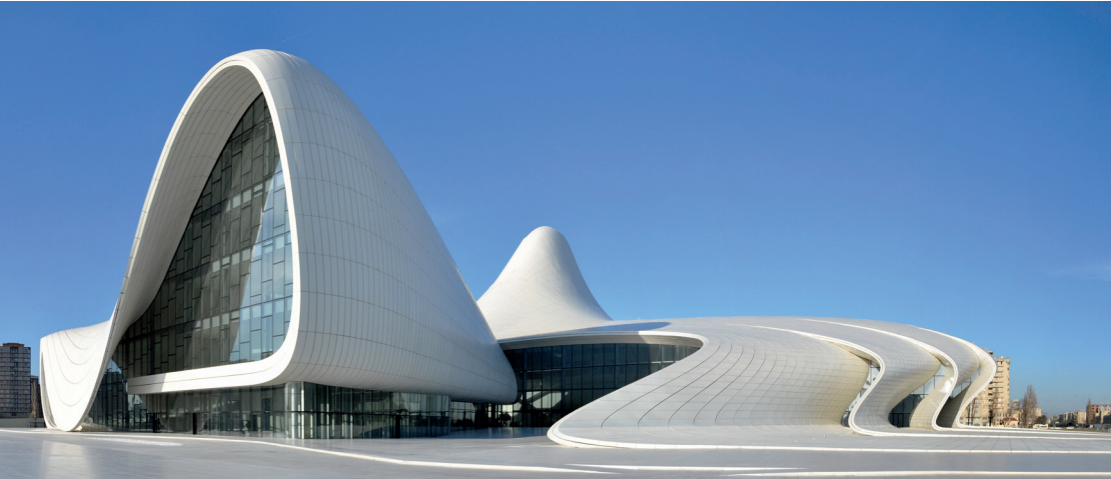
Fig. 1. Heydar Aliyev Center in Baku, Azerbaijan, 2012. Zaha Hadid Architects.
