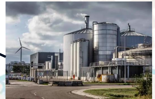
Renewi (waste composting)
