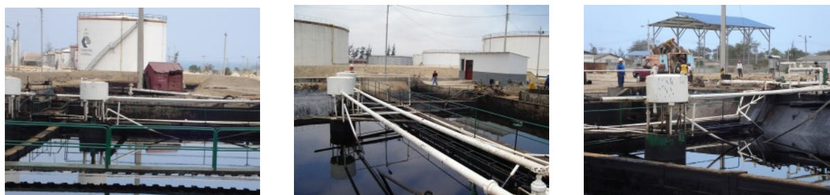
Figure 4.9: Oil collection tank API-Separator 1
