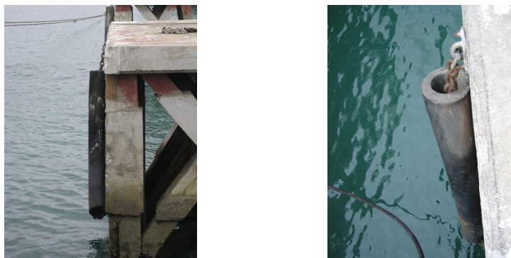
Figure 2.13: Fenders used to protect the dolphins
