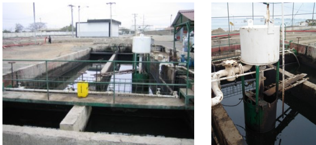
Figure 4.14: Oil collection tank API-Separator 2
