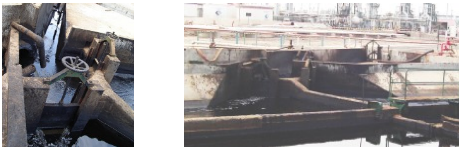
Figure 4.8: Inlet construction API-Separator 1
