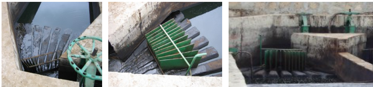
Figure 4.12: Inlet construction API-Separator 2
