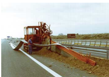
Figure 33: Installation of composite drainage as road shoulder drain
