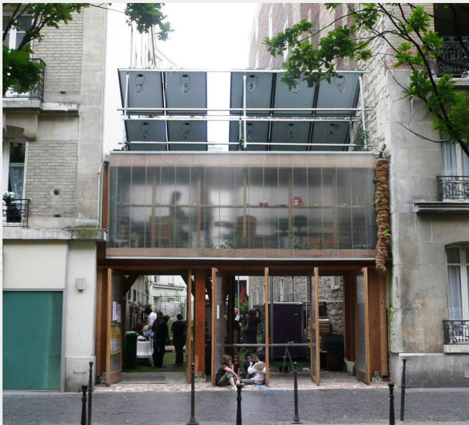
[10] The Passage 56 community Garden on a previously abandoned plot in Paris (2005)
