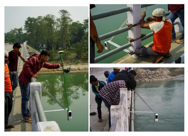
Figure 5: (left) RTK GPS is being used to get the exact elevation and coordinates of the radar gauge at GER10. (top right) Local engineer attaches the custom mount to the bridge. (bottom right) Installation of the second gauge at KAU6.
