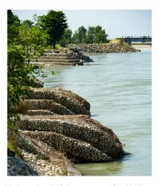
Figure 2.2: Embankment along the Kauriala branch, with failing groynes (Oct 2023).
