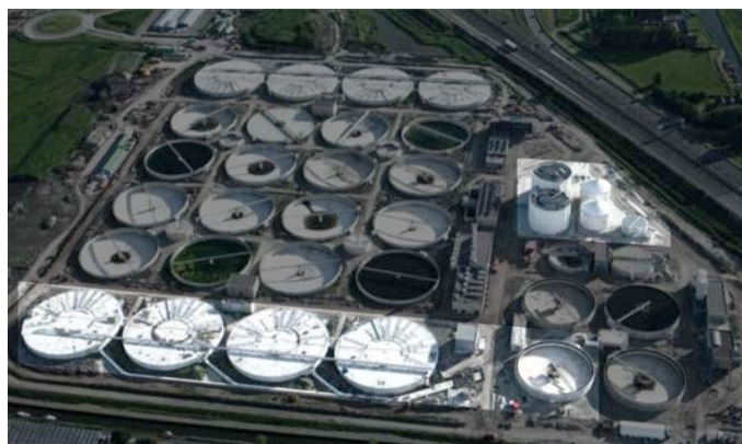
Image 7: Picture showing 75% decrease in required space by Nereda wastewater treatment system compared to CAS (own image based on xxx).
