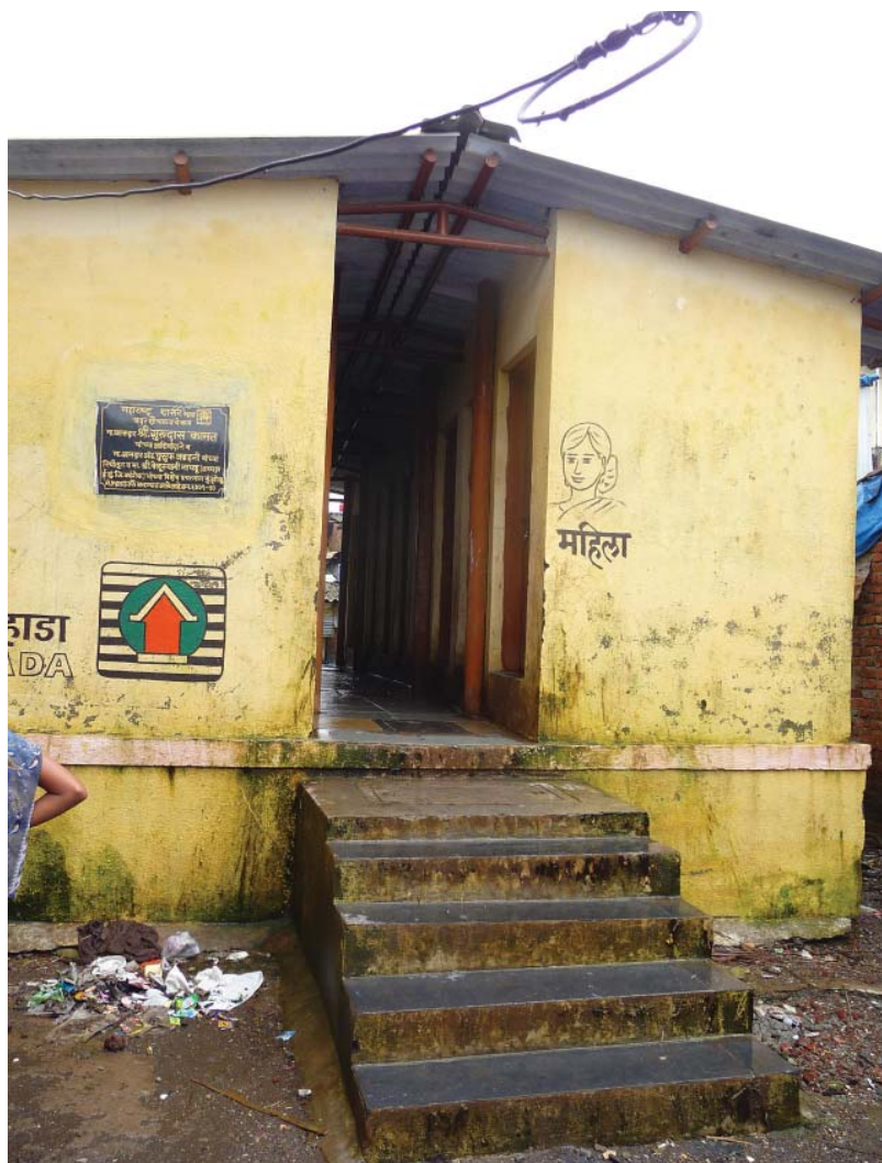
27. Basic community toilet block in Ekta Nagar
