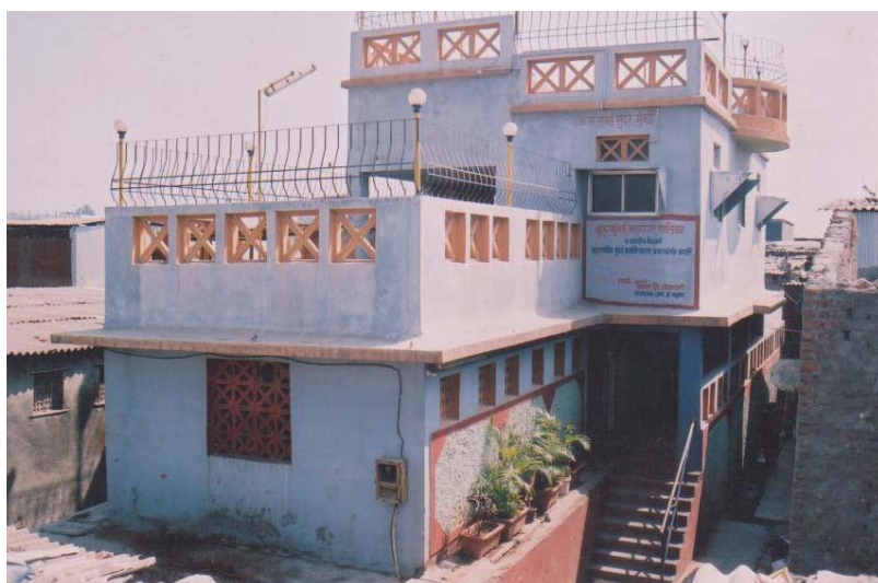
29. Baiganwadi toilet block with caretaker's house on top
