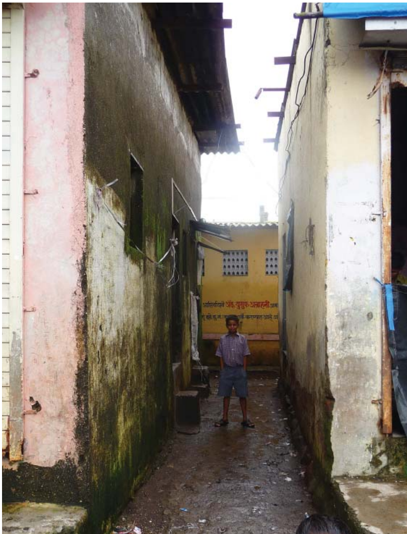
35. Access to municipal toilet block Ekta Nagar
