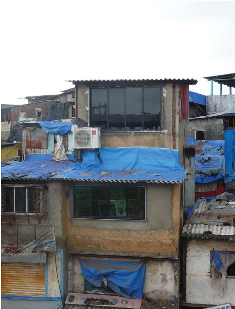
20. Air-conditioned double glazed slum house
