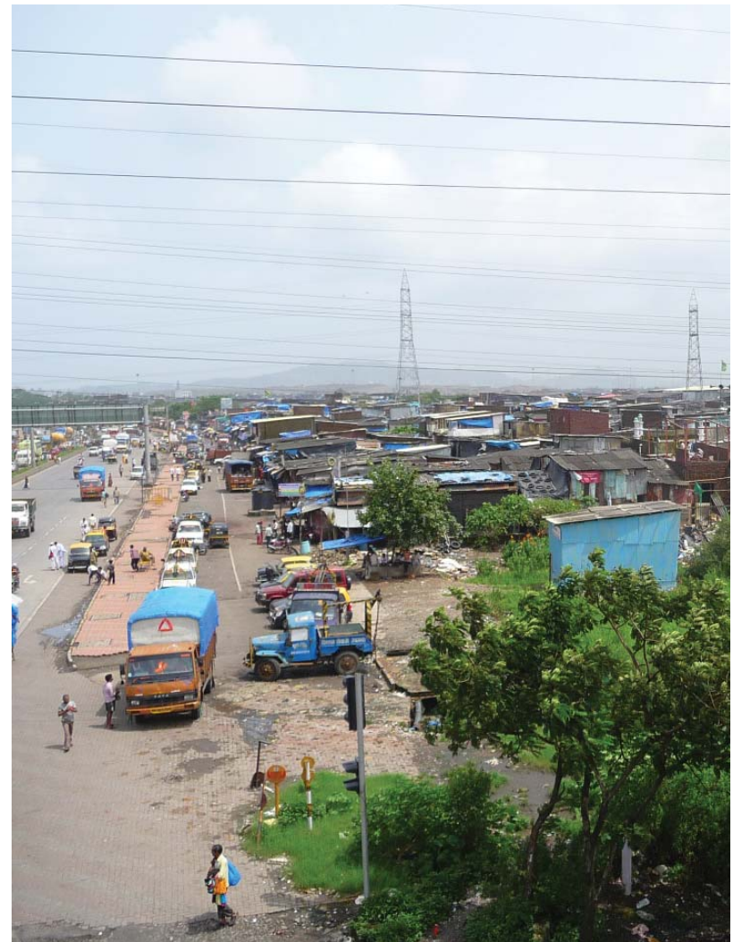
38. Entrance to Ekta Nagar along main road where men go for trade, chat and transport
