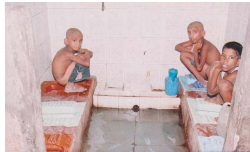
26. Children's toilet in Baiganwadi toilet block
