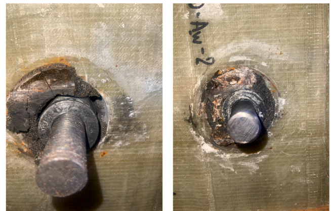
Fig. 11. Failure mode of iSRR connectors under cyclic loading after water submersion.
