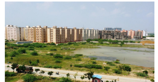
Perumbakkam Resettlement Colony (TNSCB). Source: Divya, Annie. Retrieved from https://www.cag.org.in/blogs/tn-slum-clearance-board-through-lens-cags-audit-report-part-ii .
