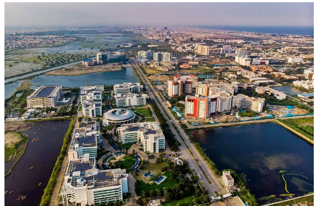
Encroachments on Pallikaranai wetland
