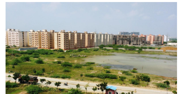
Figure 3: Divya, Annie. A view of the multistoried Perumbakkam Resettlement Colony built by Tamil Nadu Slum Clearance Board. Retrieved from https://www.cag.org.in/blogs/tn-slum-clearance-board-through-lens-cags-audit-report-part-ii .
