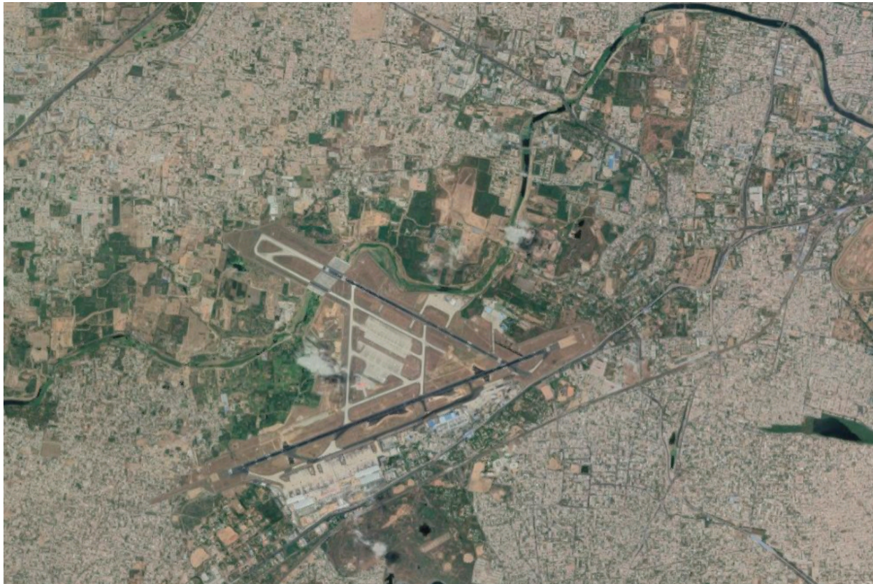
Airport built over the Adyar river
