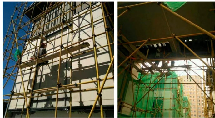
Figure 12. The installation process of insulation boards.
