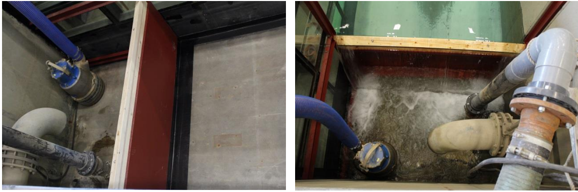
Figure 19: Weir and pumps before tests (left) and in action (right)
