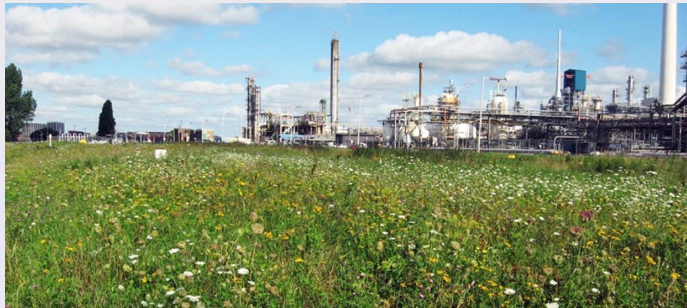
Flowerly meadow under the pylons at the port of Rotterdam Source: Making Urban Nature, (J. Vink, P. Vollaard, N. Zwarte)
