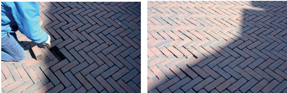
**Figure 4-5.** Case #29 has been assigned the root cause Incomplete knowledge about the interactions of SUDS with other urban systems. Due to the impact of cars as well as street sweeping, the joints of the permeable pavement bricks vanished. This decreased the overall performance of the SUDS; i.e., the stability of the road surface.
