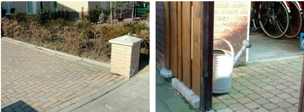
**Figure 4-1.** Two cases (#13 and #15) of technical failures in SUDS with a failing function of conveyance. Left: an obstacle interferes with the transport of water by an open gutter. Right: due to insufficient slope of the garden, the storm water flows into the shed.
