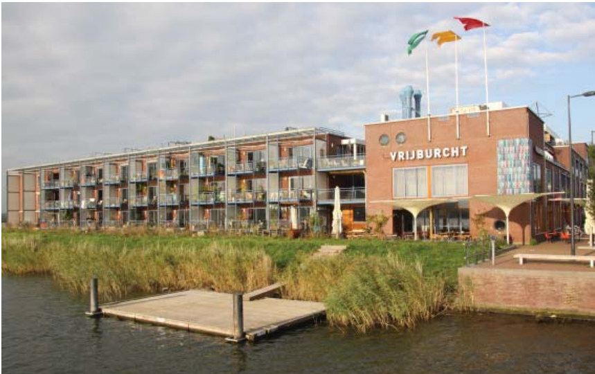
Figure 54. Vrijburcht south facade with the dock and cafe on the corner.
