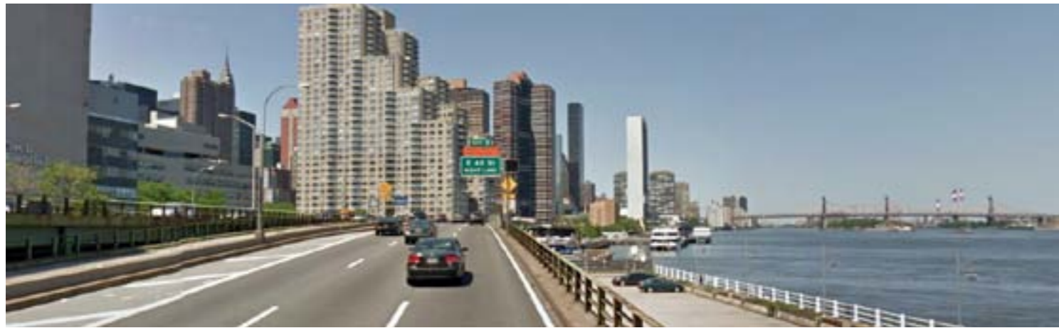
Photograph of the existing waterfront in the East side of Manhattan. There's the city, the FDR Drive and then the deck for the waterfront.
