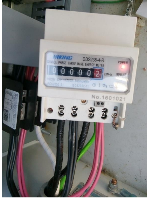
Figure 20 Installation of the electricity meter in the meter cupboard
