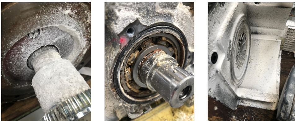
Figure 3.4: Result of blockage, Flour inside vacuum pump
