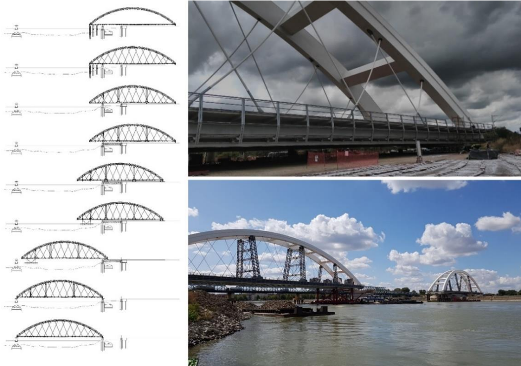
Figure 9. Launching of arch bridges over the Danube.
