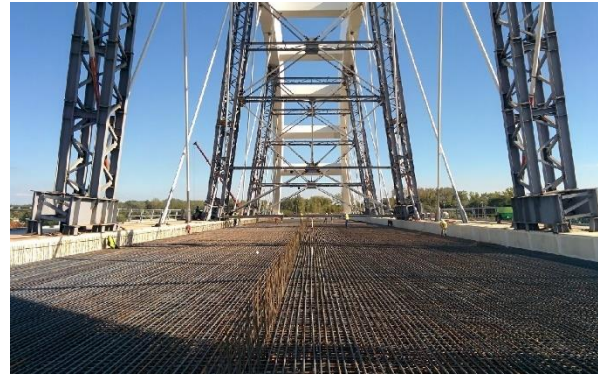
Deck reinforcement installation. The temporary columns for launching are still on place.
