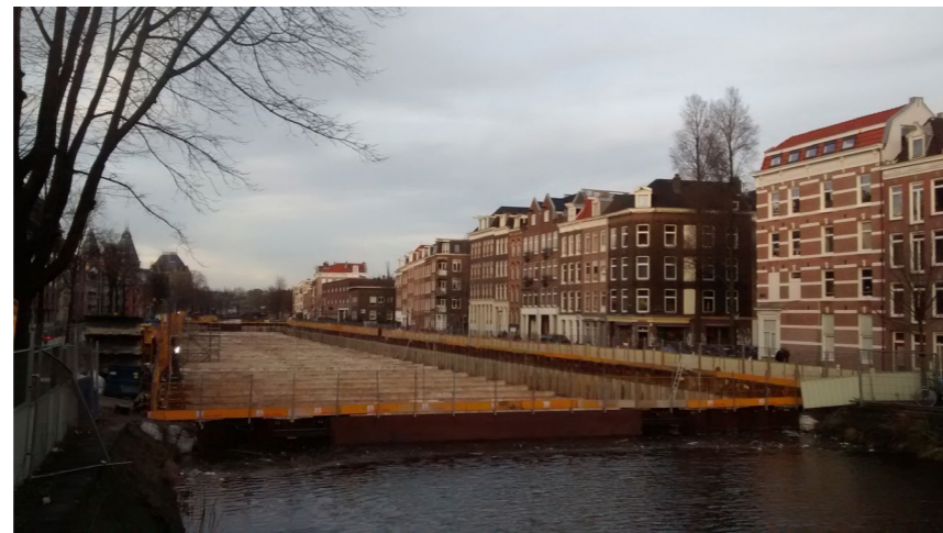
61 The parking garage under the Boerenwetering canal under construction.
