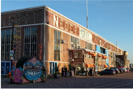
Exterior of the warehouse at the NDSM Wharf East area.
