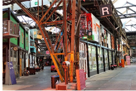
The "Art City" inside the warehouse: a steel frame where 80 artists constructed their own studios.
