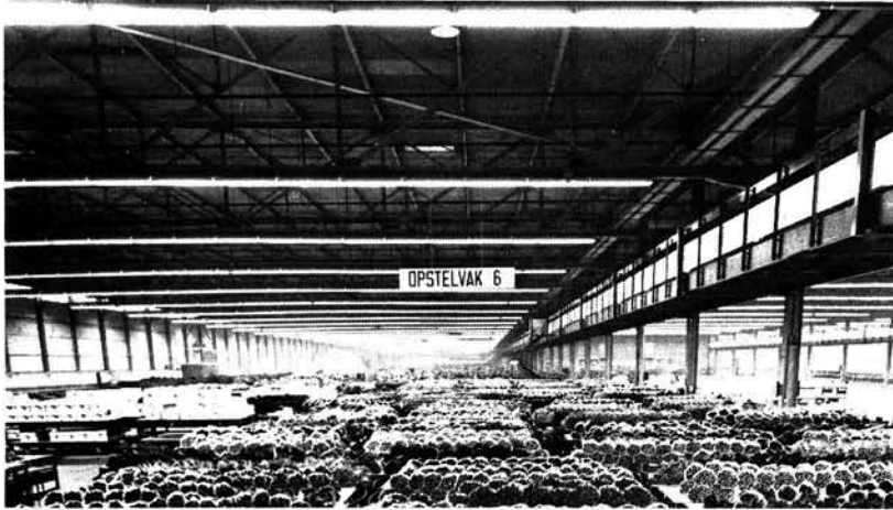
Figure 6.6.1. Typical example of application of hot-dip galvanized steel: nearly 10.000 tons have been used for the enormous halls of the Aalsmeer flower market.
