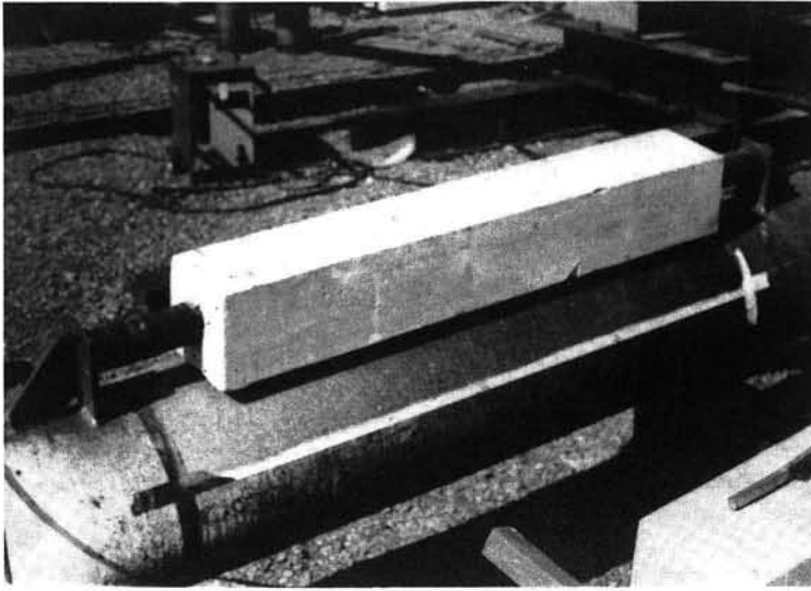
Figure 6.5.3. Part of off-shore drilling platform with aluminium sacrificial anode (Vandervelde Protection, Rijswijk, Netherlands).
