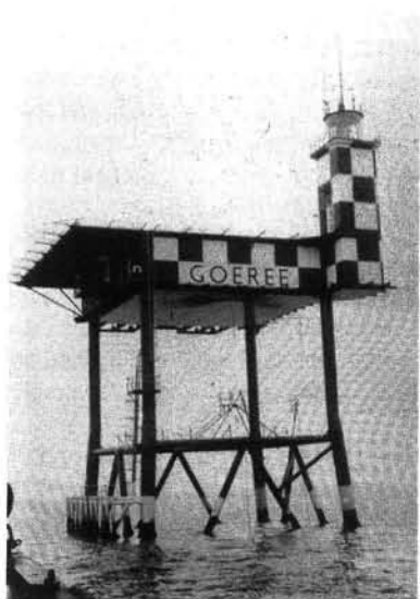
Figure 6.6.2. Light platform "Goeree" with vitreous enamel panels which are still completely bright after 10 years (Ferro (Holland) B.V., Rotterdam).
