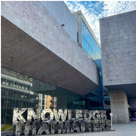
20% in front of the Via Roentgen Building
