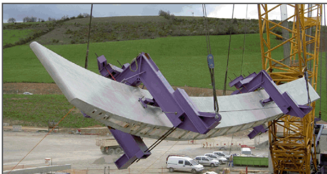
Figure 4.17: Millau toll gate element. UHPC is positioned at the outside. Picture from Servant [53].
