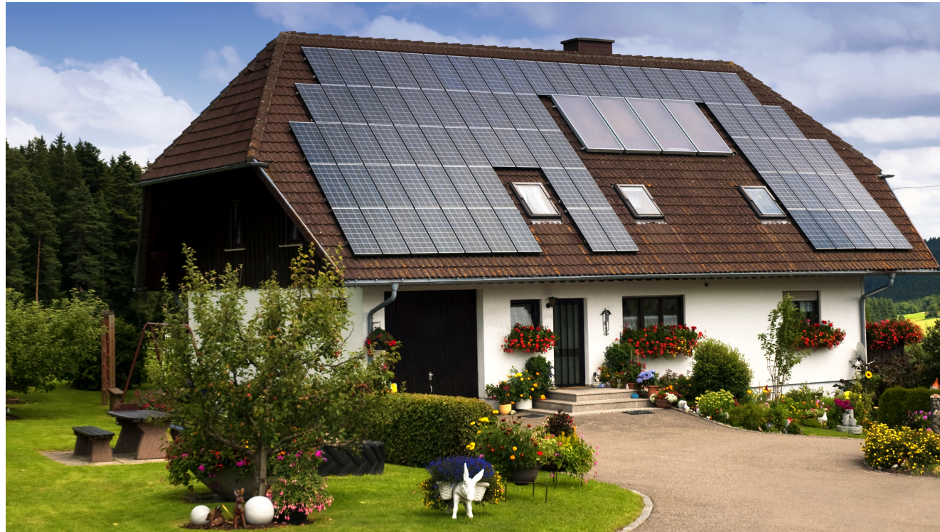
Image: courtesy of Modernize
