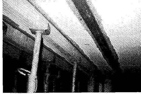
Fig. 1.6 Removal of temporary supports; floor strengthened with steel plates
