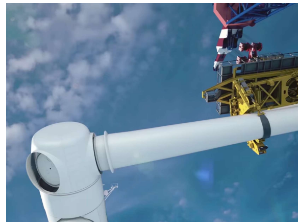
(d) Mating phase: The blade is slowly moved towards the hub
