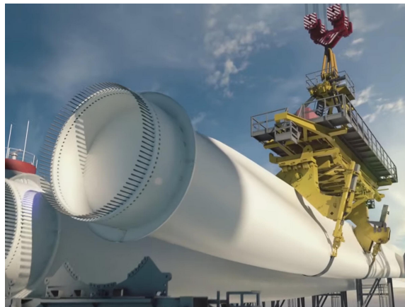
(a) Crane lifting a blade from the storage racks used for sea fastening
