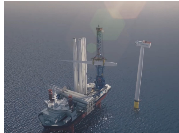
(b) Lifting phase: Blade lifted from deck and moved towards the hub
