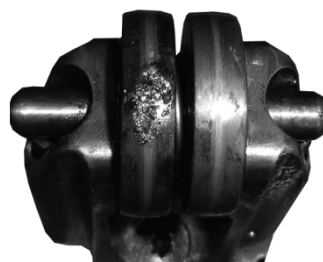
Figure 2.11: Left Showing extreme pitting on the stator contact surface, Right showing: Change-over selector stator roller contacts are damaged in the advanced stage of the long-term effect [3].
