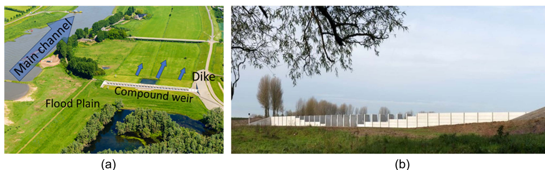
Fig. 1. (a) Aerial view of the compound weir located at the right bank flood plain of the Pannerden bifurcation in the Netherlands (image courtesy of Rijkswaterstaat, The Netherlands); and (b) the compound weir closer view from upstream, Rijnwaardense Uiterwaarden (n.d.) (image courtesy of Marc Plum).
