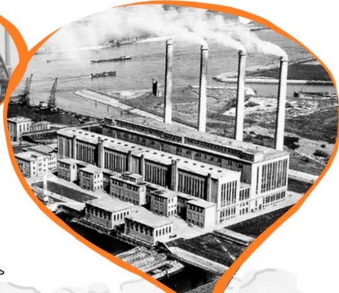
Merwede power plant
