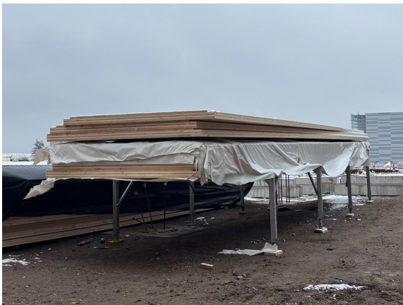
(a) CLT panels stored outdoors under temporary protection.
