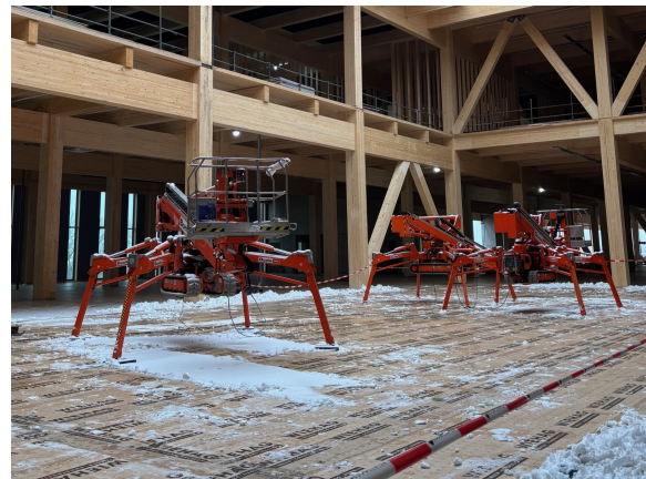
(b) CLT floor panels during erection.
