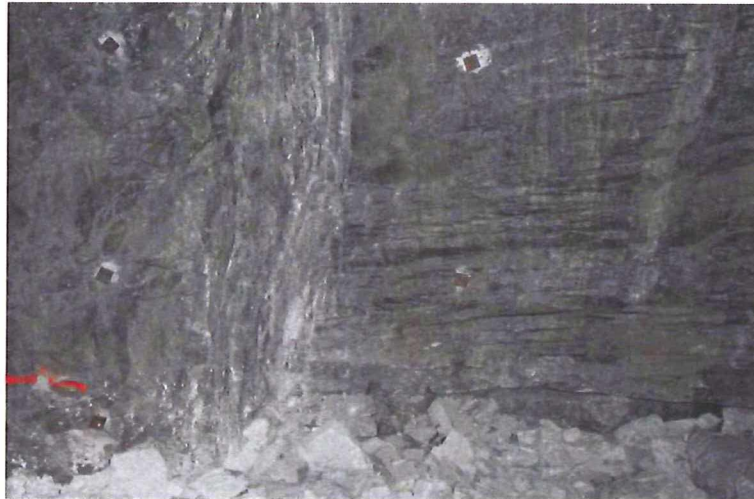
Figure 5.12: Horizontal stress induced fractures in the ore up to the footwall contact. (Nyström, 2008)
