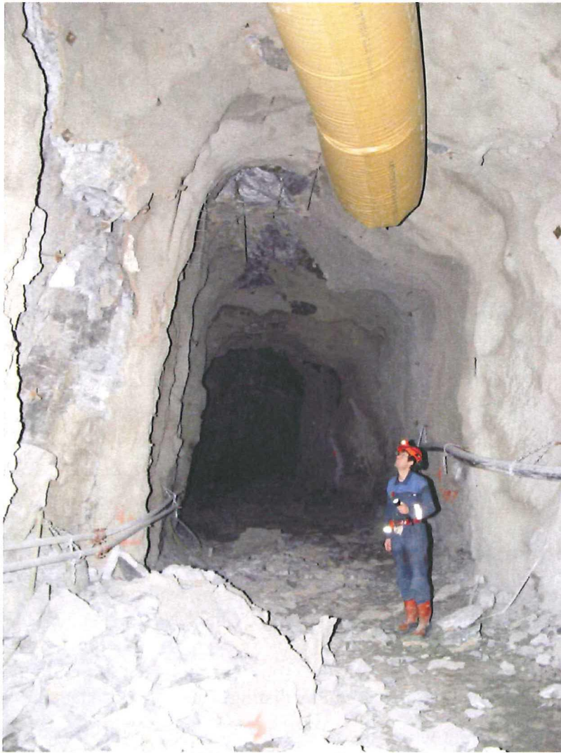
Figure 10.14: Displaced material from the wall and along the centre of the back further down the drift. Anders can, in this case, be used as a scale. (Nyström, 2008)
